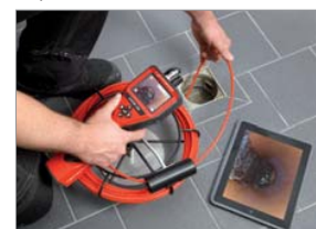
Inspection of floor drains
